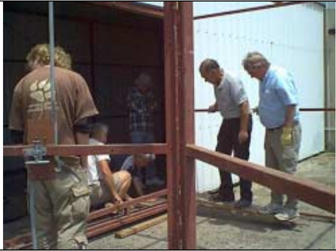
Ryan and Larry lend their weight on a pry bar to adjust the hangar frame.
